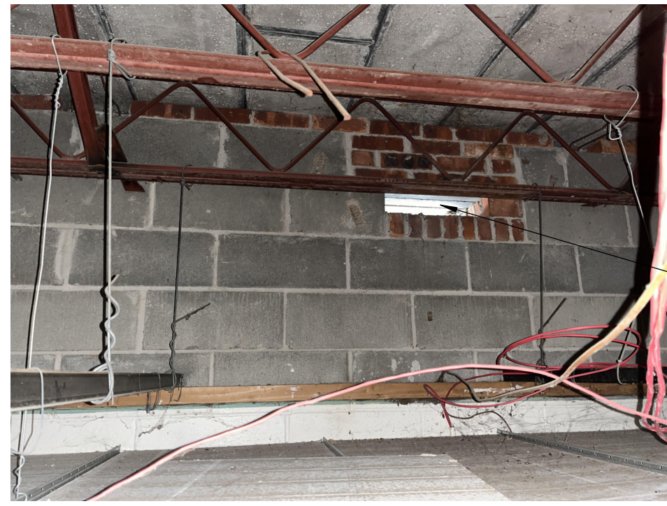
5 EXISTING EXTERIOR WALL OPENING SCALE: NOT TO SCALE
