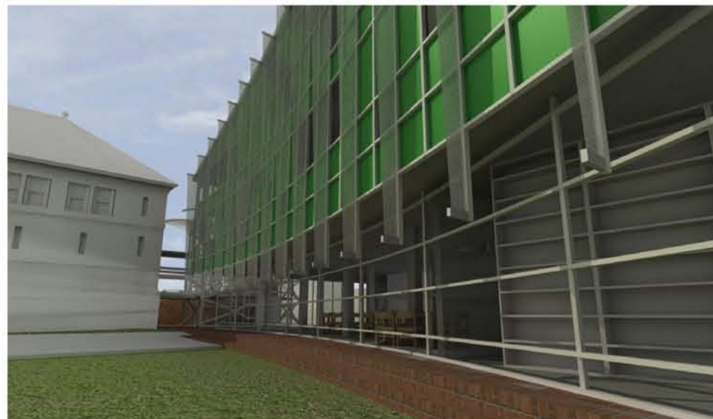
The north-east façade utilizes vertical shading devices to minimize heat gain through the curtain wall. The addition hovers next to the massive form of the existing library tied to it by a transparent glass bridge on the second story.
