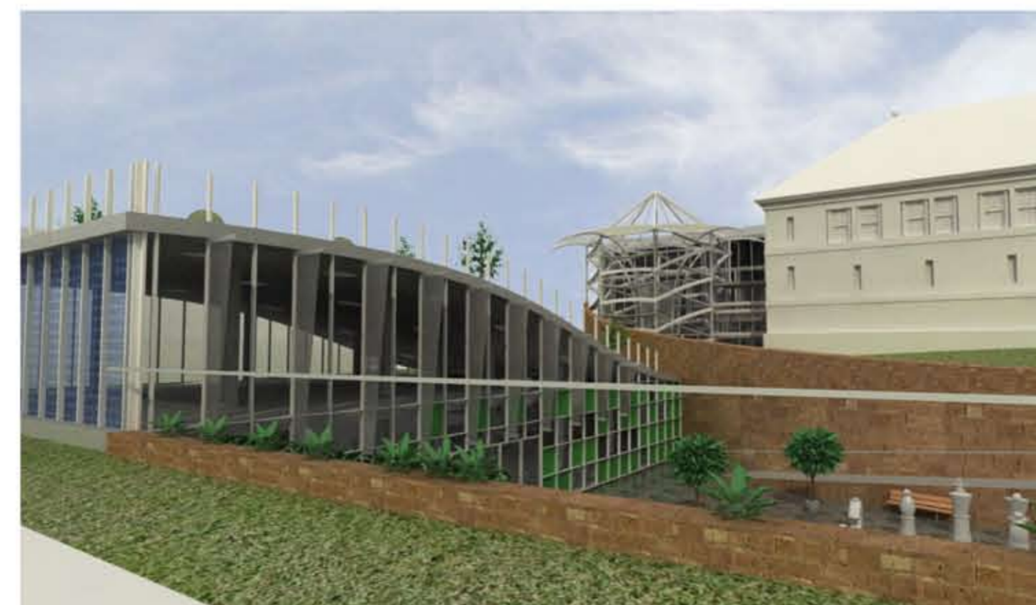
Pedestrians walking by have a unique vantage point of the “digital wall” which displays news and community events. Vertical fins shade the eastern façade and add character. Solar panels on south facade take advantage of alternative energy solutions.
