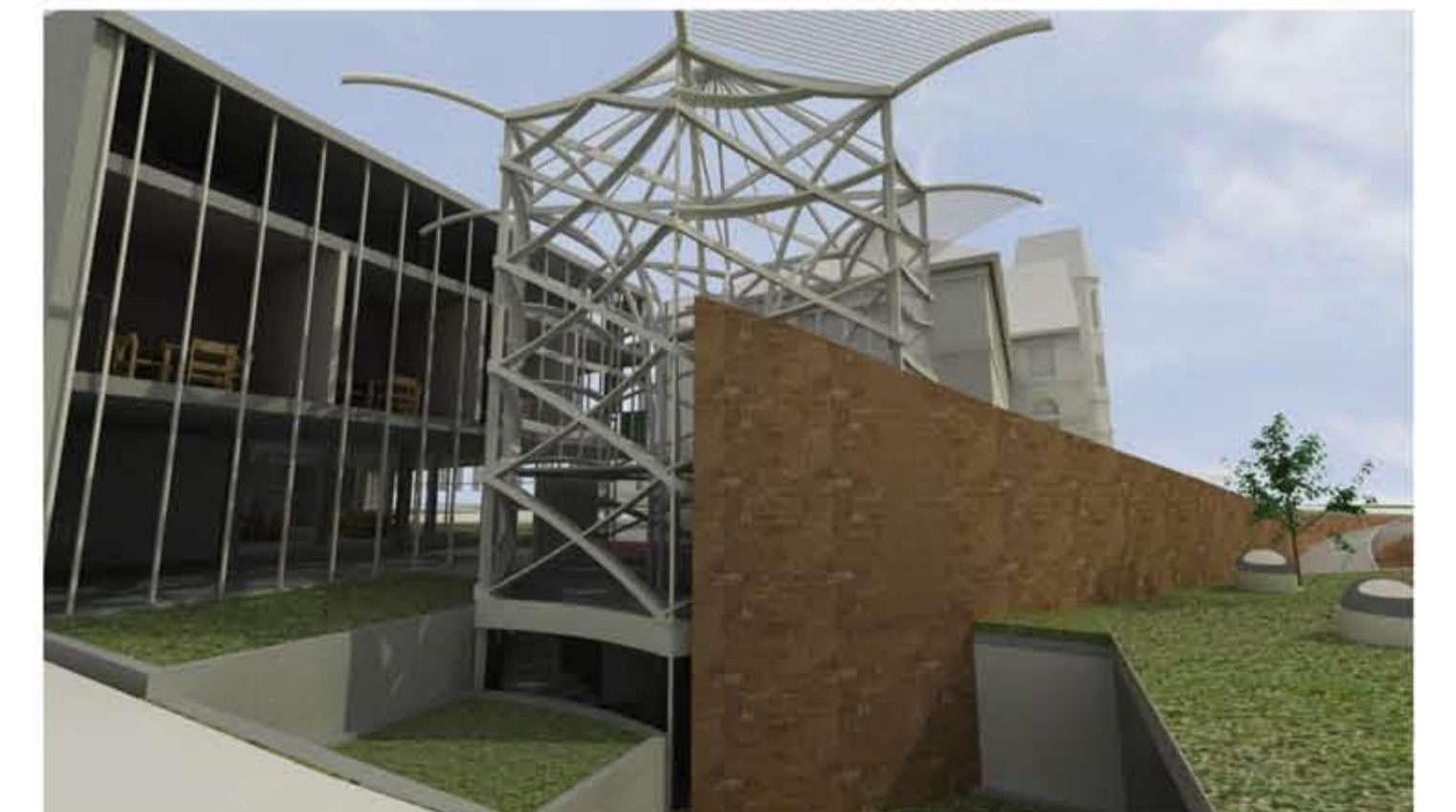
The rusticated stone wall wraps around the rear of the circulation core to translate the materiality of the existing building into the new addition. Stepped courtyards allow daylight
