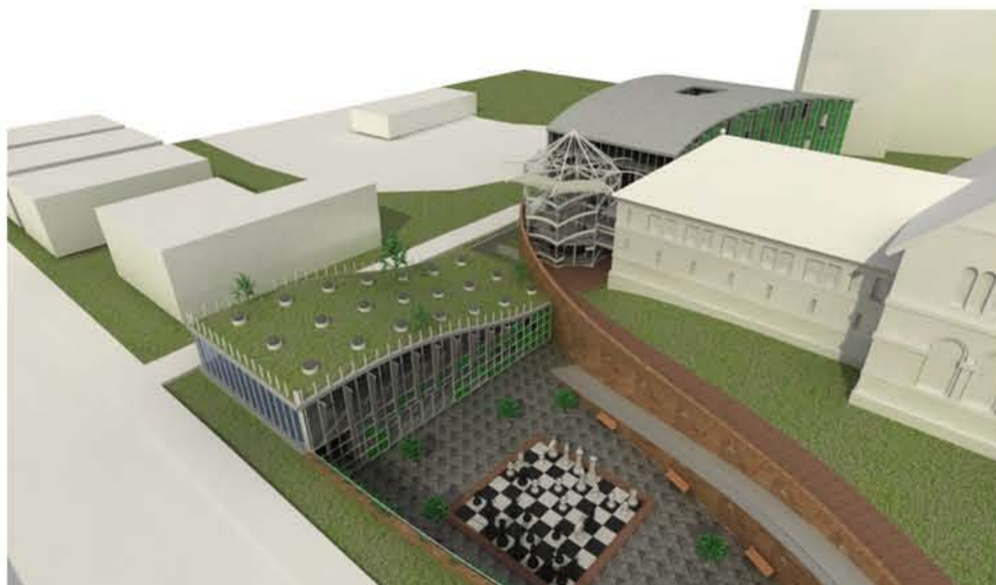
An aerial perspective of the site highlights the below-grade public courtyard and the circulation core which ties the new addition to the existing building. Solar tubes for daylighting extend from the undulating vegetated roof above the community space.
