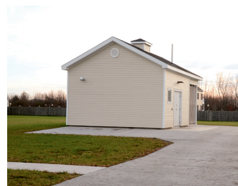
West Washington St. lift station with porous concrete pavement
